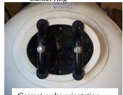
Correct yoke orientation
