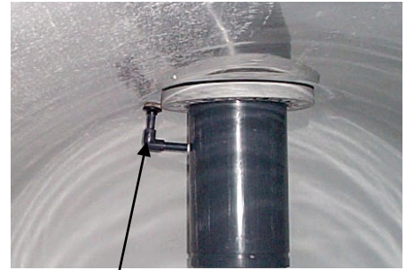
Automatic Air Relief Assembly
