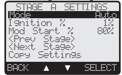
Modulating Boiler Stage Menu
